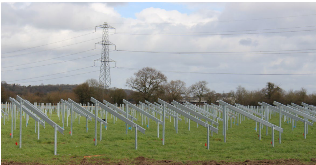
Plate 11c: Installation of Mounting Structures (3 of 4)
