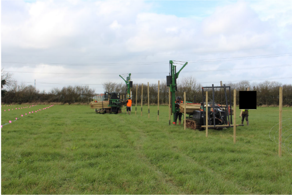
Plate 8: Establishment of Site fencing
