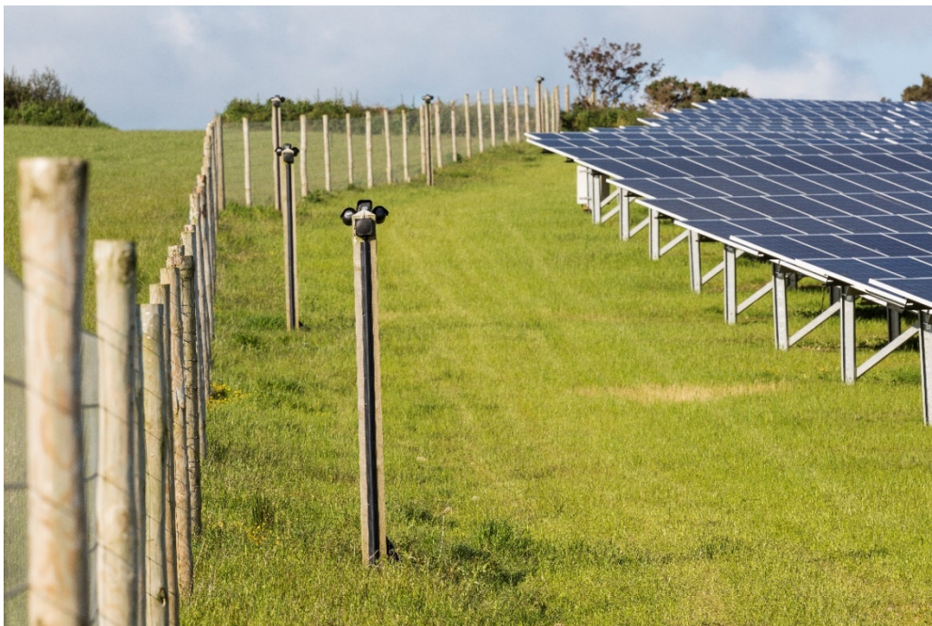
Plate 5: Example of security fencing and monitoring cameras
