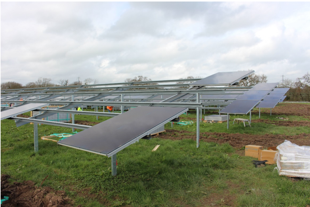
Plate 12: Mounting of PV Modules
