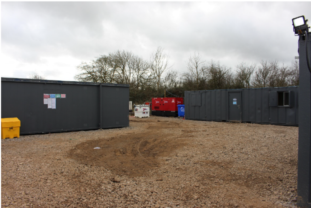
Plate 9: Establishment of the temporary construction compound(s)
